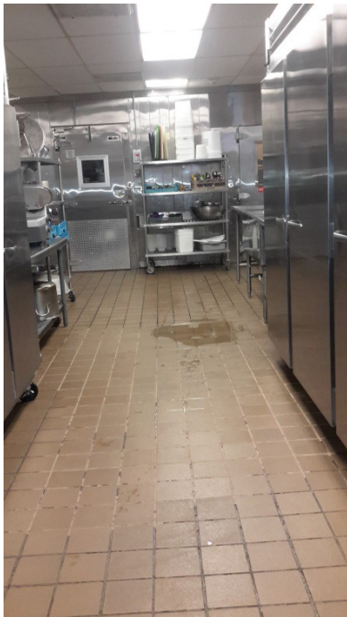
Reach in refrigerators on each Side of aisle
