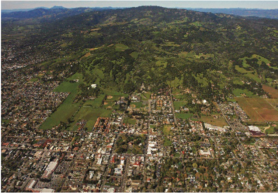
Aerial View of Sonoma County.
