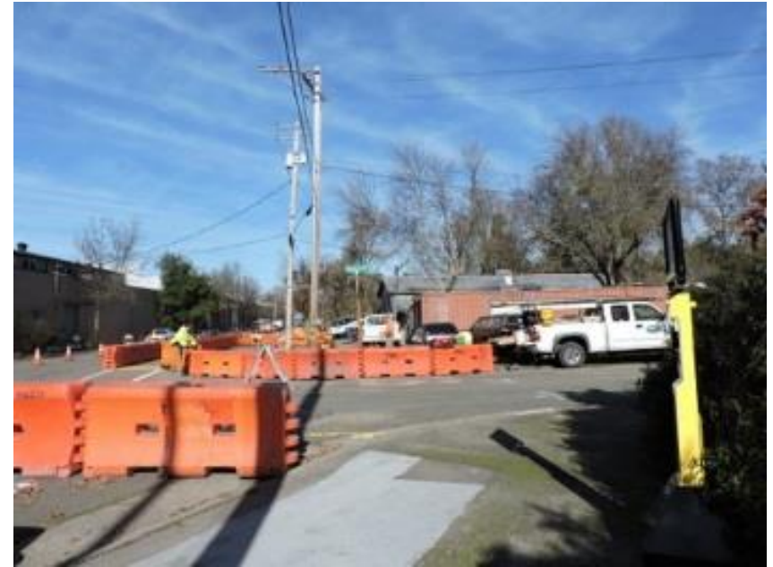
Graton Accessibility Improvements Temporary barricades and audible devices during construction
