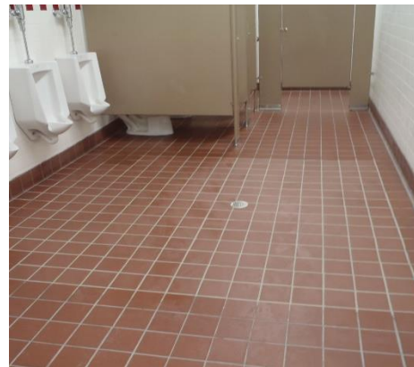
Hall of Flowers Toilet Room Floor Level (16/17)
